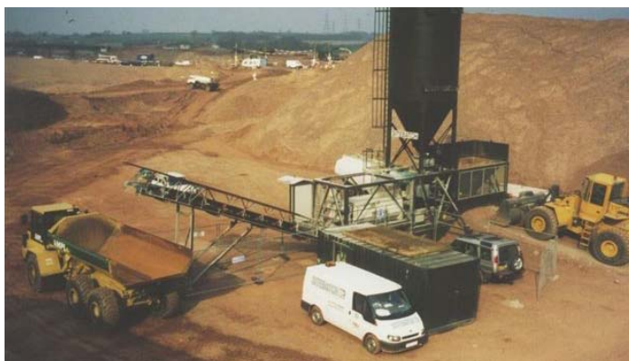
Production facilities of HBM mixtures
