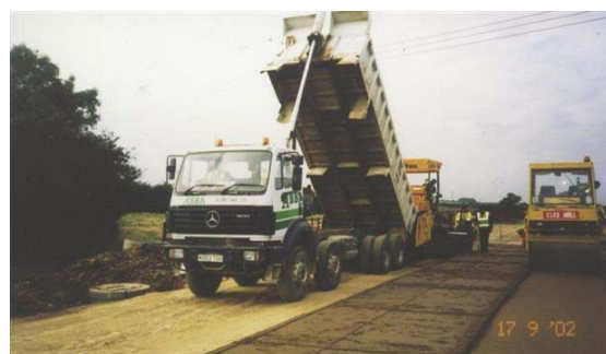
Laying of a major road with HBM mixture containing RSA.
