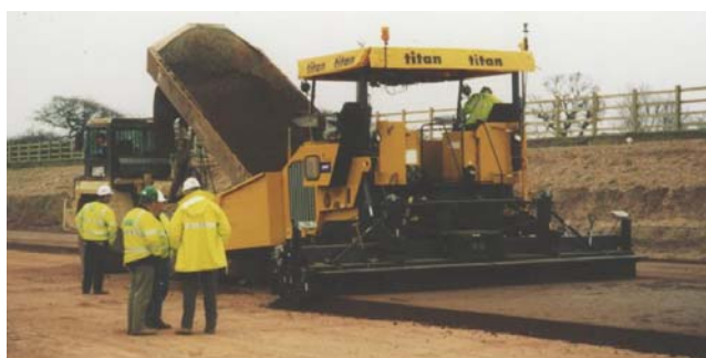
Laying of a major road with HBM mixture containing RSA.
