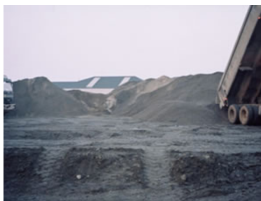
Stockpile of HBM mixtures
